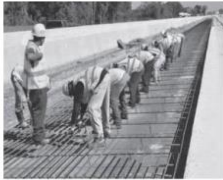
Placing reinforcement
