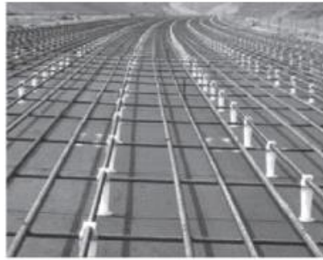
Reinforcement ready for concrete
