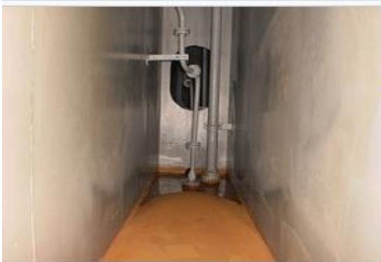
Inside of a cofferdam on a vessel
